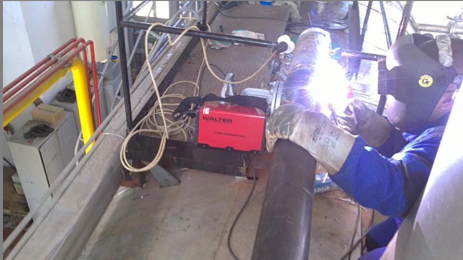
**100% KVALITETAN ZAVAR BAZICNOM I CELULOZNOM ELEKTRODOM DO 3.25MM.**
